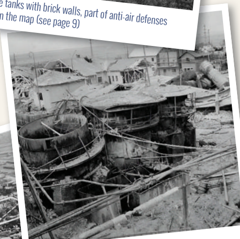
Damages to Vega Refinery after the Allied raids in May-August 1944
